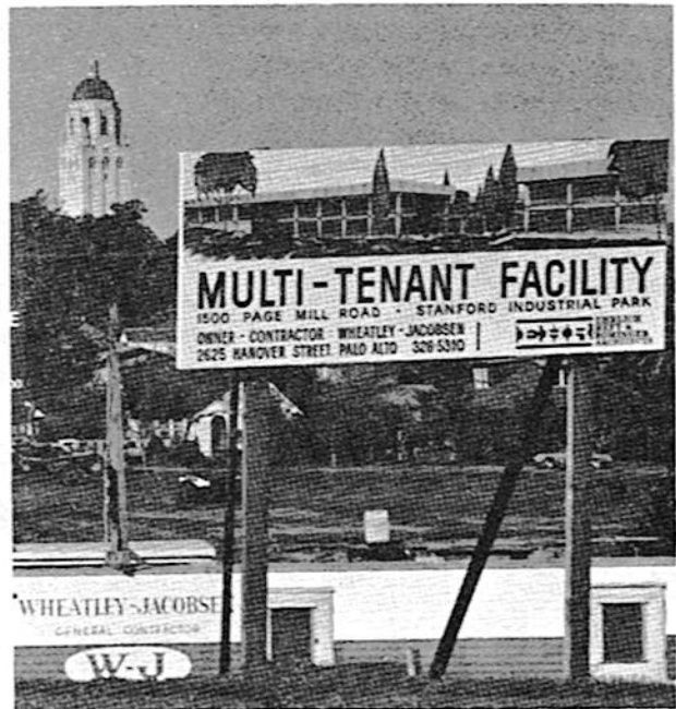
Jack Wheatley splits his time between sitting on Palo Alto's City Council and supervising construction in the Industrial Park.
