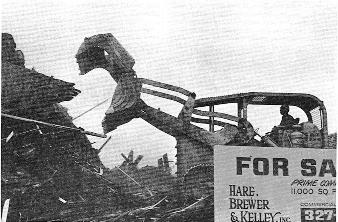
A large realtor and a bulldozer continue the Palo Alto pattern of demolishing old, low-rent homes.
